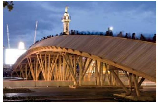
The footbridge designed by the architect Kawamata between the Place des Quinconces and the riverside in Bordeaux was built using Everad polyurethane adhesive
