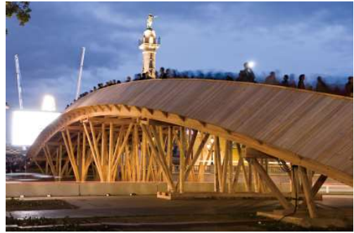
The footbridge designed by the architect Kawamata between the Place des Quinconces and the riverside in Bordeaux was built using Everad polyurethane adhesive
